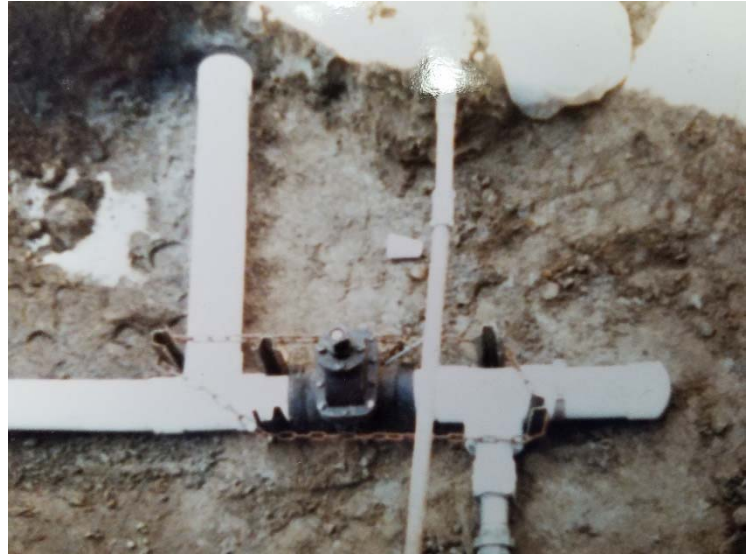
PHOTO 1 - PVC WATER MAIN (ROUTE 9 SOUTH)
